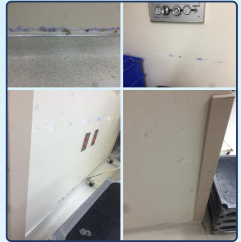
Examples of most OR wall surfaces after a short period of time. This example shows OR's that are only 2 years old.
